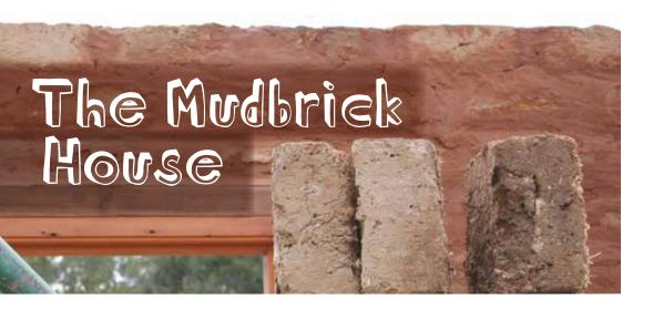
There are enormous advantages to building your home using traditional Mudbricks. The environmental benefits begin with utilising the dirt from your own house excavations, mixing it with water and straw, and drying the moulded brick in the sun. This provides a low-embodied energy wall material, and presents a warm, inviting look to your home.
